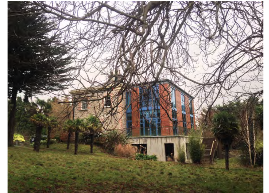
Cedar Mount House, Side view, existing
