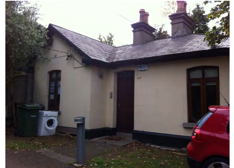
Gate Lodge West, existing
