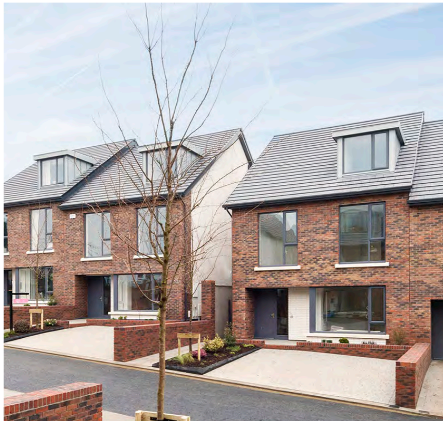
Completed Houses in Phase 1, Knockrabo
